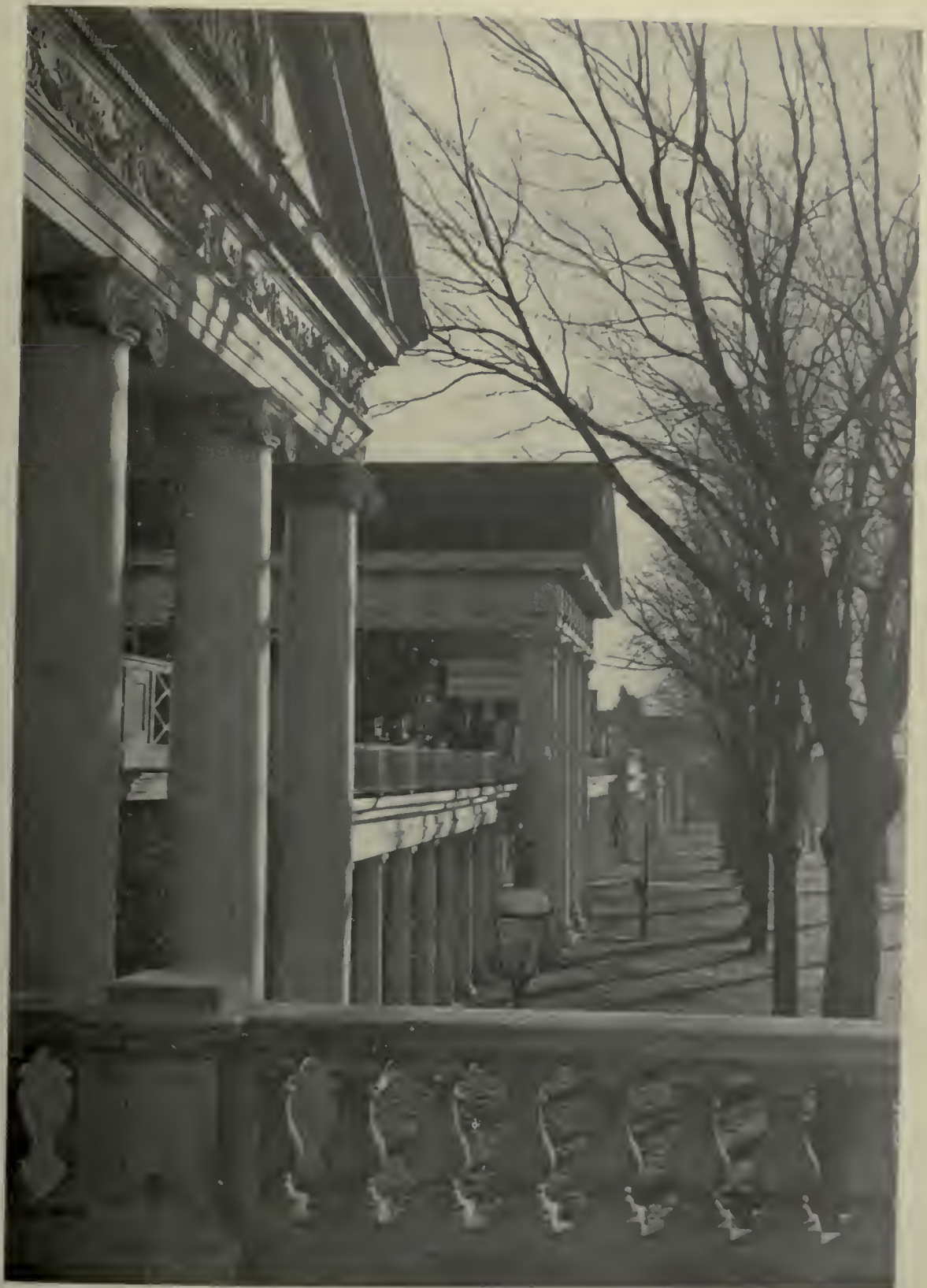
East Lawn From Terrace Over Administration Offices.
